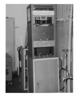
This is the Alexian Brothers site, (inside the equipment shack on the roof). The 440 repeater, W6UU, is in the cabinet on top, the BBS is in the lower cabinet. (The cabinet in back is a pager.) The angle bracket bracing is visible at the right of the repeater cabinet. It's bolted to a metal rail (part of the structure) and both cabinets are bolted together.
